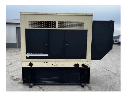
\_\_80 KW KOHLER GENSET, ENCLOSED, SOUND ATTENUATED, WITH JOHN DEERE ENGINE, YEAR - 2007, 734 HOURS, US EPA TIER 3
