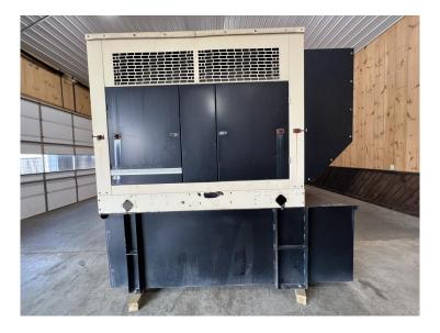
Fuel Diesel Year 2007 Voltage 120/240 Volts Hours 148 Hours Phase 1 Phase Make Kohler Model 60REOZJB Serial 2142925 Hertz 60 Hz Wires 4 Lead Kilo Watts 60 kW Mounted Skid Mounted Fuel Tank Base Fuel Tank Enclosure Sounded Attenuated Enclosed Enclosed Length 111" Width 41" Height 108" Weight 4500 lbs Condition Well Maint. Unit, Tested, Serviced, Ready to go Circuit Breaker Yes
